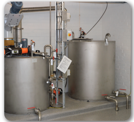
Inside the water station, sodium is added to raise the water's pH.
