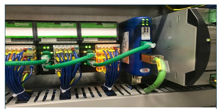
communication standard the devices use, the Communicator will enable them to communicate with our PLC anyway. Furthermore, we can now choose different PLCs to suit a specific packaging machine since the Anybus Communicator handles most network standards on the market."
